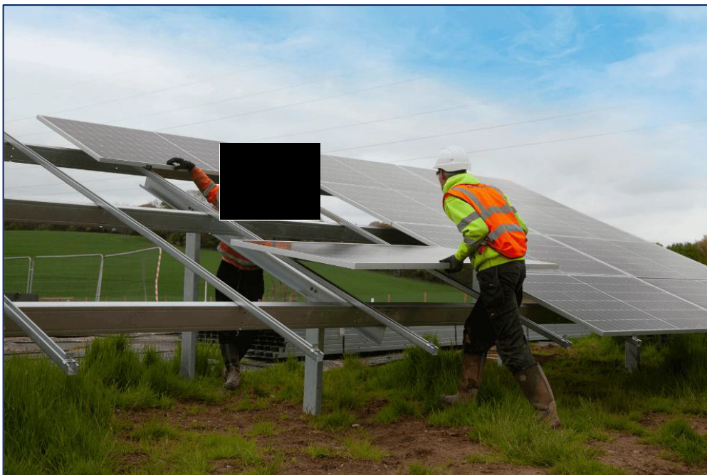
Plate 12-24 PV module installation (Ref. 12-16)
